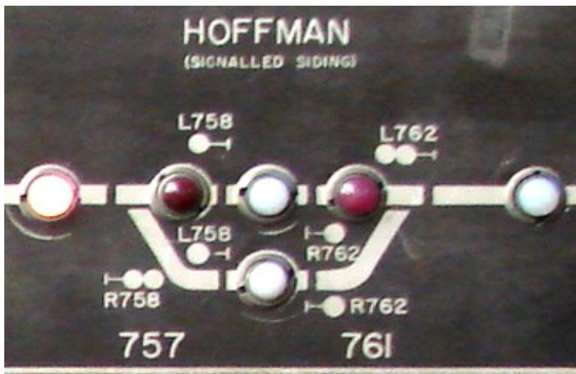
NC. This panel is now located at the NC Transportation Museum, Spencer, NC.
